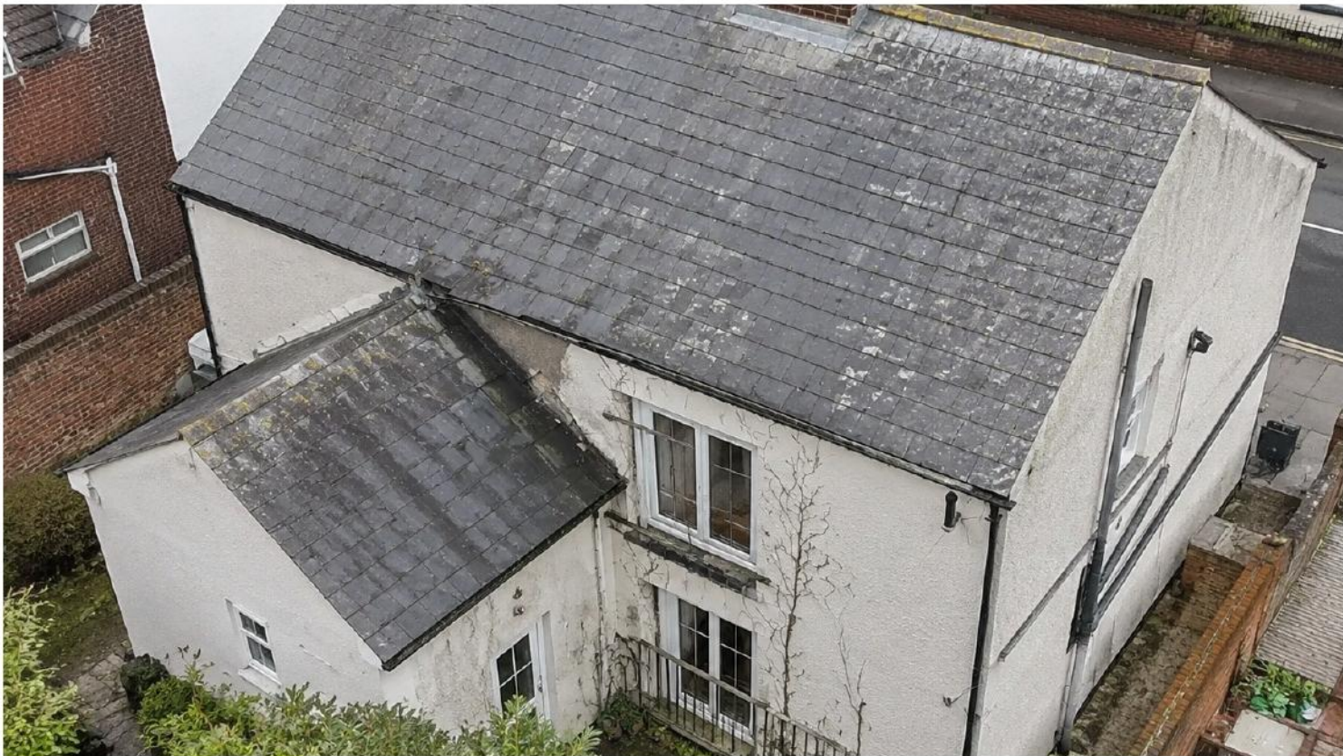
IMG-0001 • Rear oblique property overview
