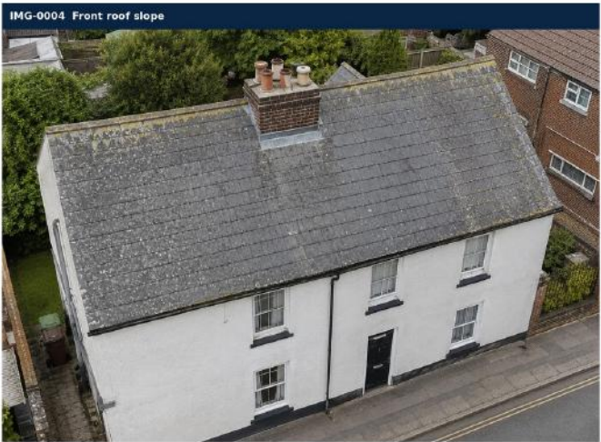
IMG-0004 • Front slope
