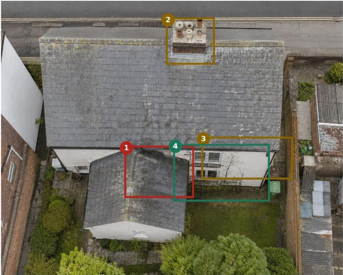
IMG-0002 • Near-vertical roof plan with finding locations
