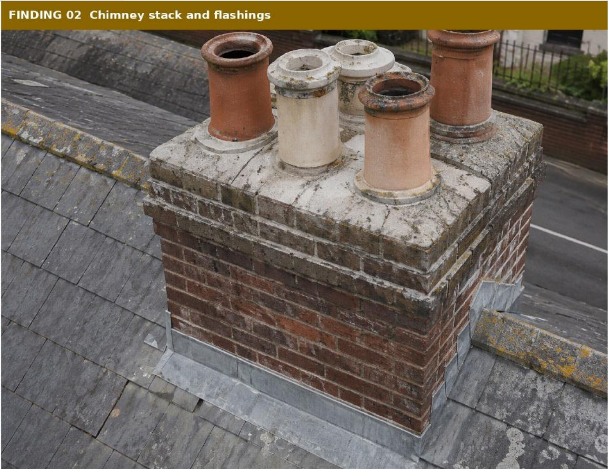
IMG-0005 • Chimney detail
